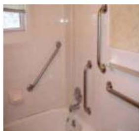
Fig. 6.1: Grab bars in side bathroom
